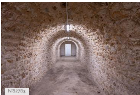
Fort de Saint-Cyr - Arched rooms
