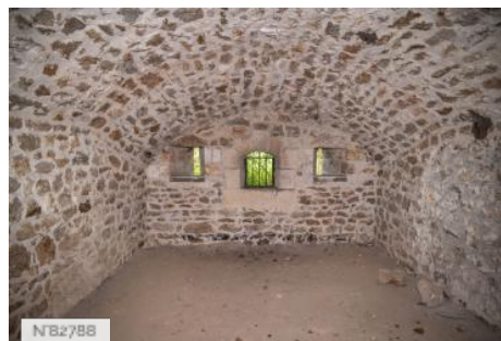
Fort de Saint-Cyr - Fire station room
