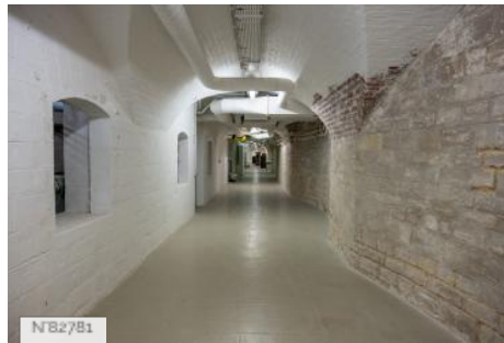
Fort de Saint-Cyr - Interior circulation
