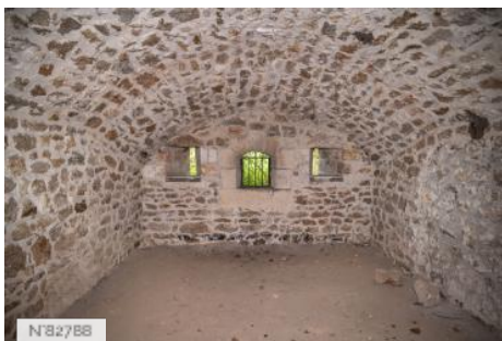
Fort de Saint-Cyr - Fire station room
