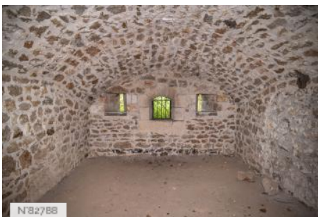
Fort de Saint-Cyr - Fire station room
