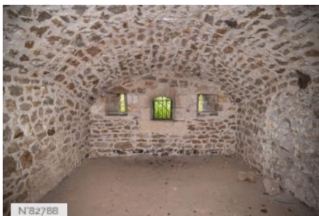
Fort de Saint-Cyr - Fire station room
