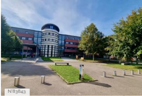
Former Nursing Training Institute - Dieppe Hospital Center
