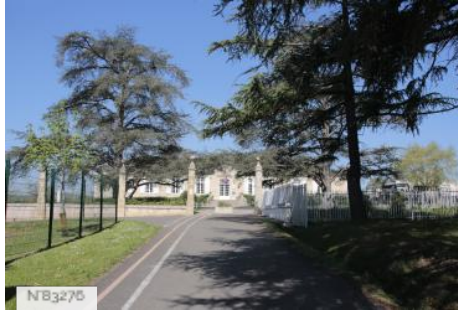
Beaulieu Lavacant highschool - Beaulieu site - Outside
