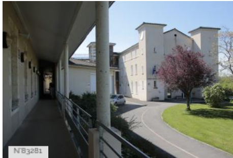
Beaulieu Lavacant highschool - Lavacant site - Outside
