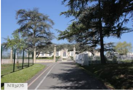
Beaulieu Lavacant highschool - Beaulieu site - Outside
