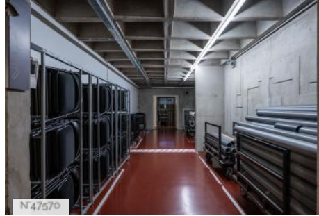
Centre National de la Danse underground parts
