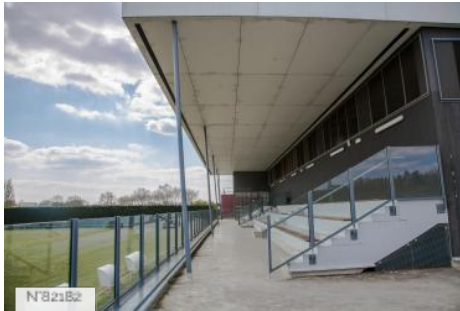
City of Evry-Courcouronnes - Lake sports complex - Outdoor bleachers
