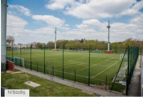
City of Evry-Courcouronnes - Lake sports complex - Artificial turf field
