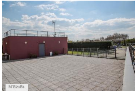
City of Evry-Courcouronnes - Lake sports complex - Terrace
