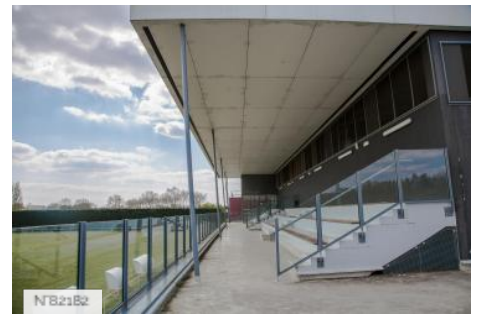
N'82182 City of Evry-Courcouronnes - Lake sports complex - Outdoor bleachers
