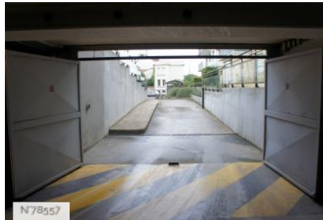
City of Nogent-sur-Marne - Municipal Technical Center - Parking lot
