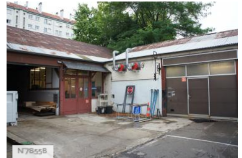
City of Nogent-sur-Marne - Municipal Technical Center - Garage
