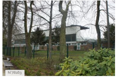
City of Nogent-sur-Marne - Stadium / Sport field / changing rooms
