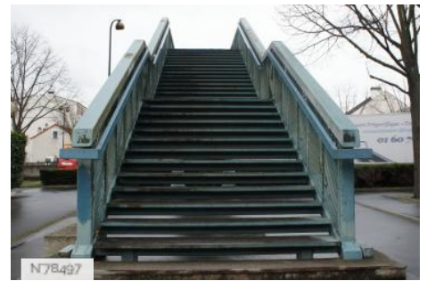
N78497 City of Nogent-sur-Marne - Hoche footbridge
