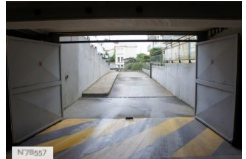
City of Nogent-sur-Marne - Municipal Technical Center - Parking lot
