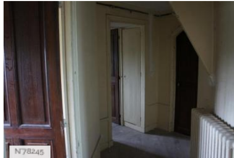
N78245 City of Les Mureaux - House of Oseraie - Attics
