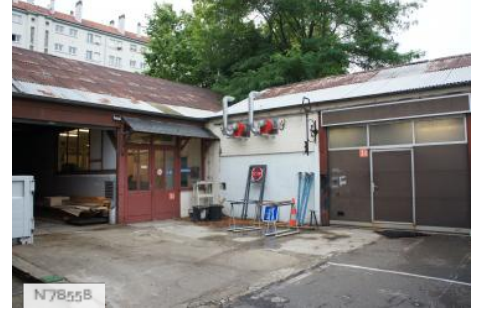
City of Nogent-sur-Marne - Municipal Technical Center - Garage
