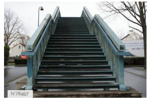
N78497 City of Nogent-sur-Marne - Hoche footbridge
