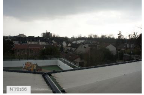
City of Nogent-sur-Marne - Leonard de Vinci School - Terrace
