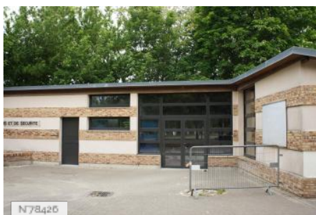
N78426 Ile de Loisirs Cergy Pontoise - First-aid post
