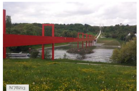
N78213 Ile de Loisirs Cergy Pontoise - Bridges
