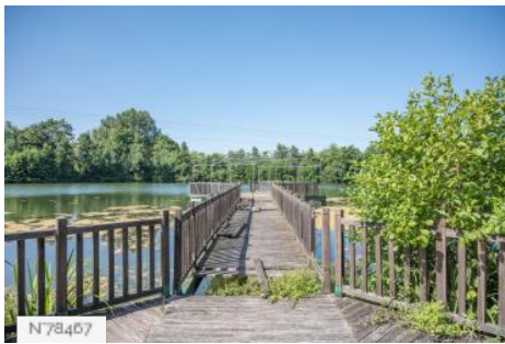
N78457 Ile de Loisirs Cergy Pontoise - Fishing pontoon area
