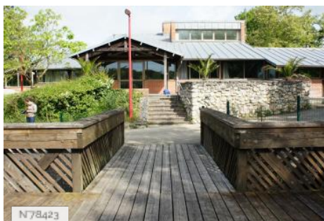
N78423 Ile de Loisirs Cergy Pontoise - Reception Hall
