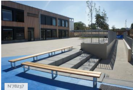
N78237 City of Les Mureaux - The Pole Moliere - Primary School
