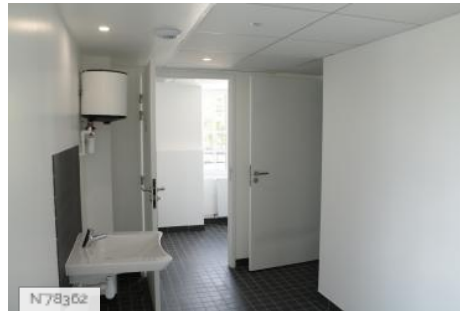
Fontenay-aux-Roses city - Music conservatory/Bathrooms
