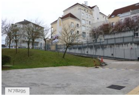
Melun Courthouse - Parking
