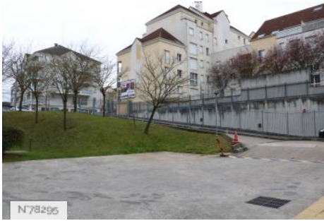
Melun Courthouse - Parking
