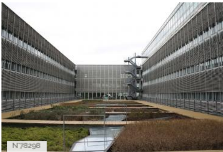
Melun Courthouse - Patio
