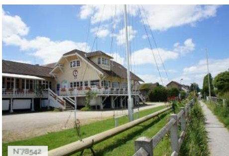
Ville des Mureaux - The Circle of the Sail of Paris
