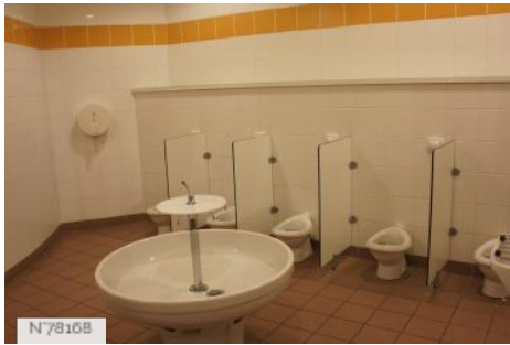
City of Nogent-sur-Marne - Leonard de Vinci School - Toilets
