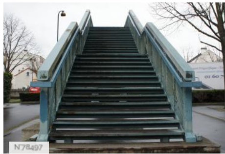
N78497 City of Nogent-sur-Marne - Hoche footbridge
