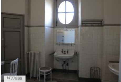
Grosbois estate - Bathroom
