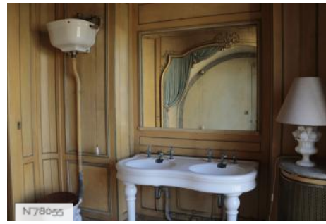
Grosbois estate - Bathroom
