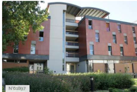
CIUP Lilas Dormitory - Cafeteria
