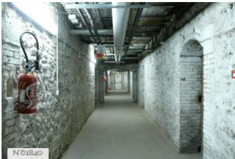
Saint Philippe Educationnal village - Cellars and undergrounds
