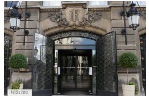
City of Vincennes - City hall - Outside
