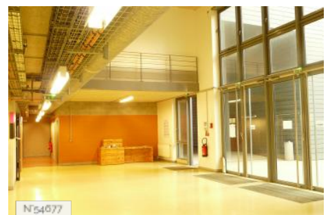
Université Paris Diderot Paris 7 - Condorcet building entrance hall
