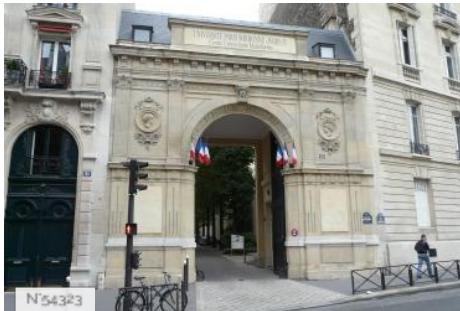
Centre Malesherbes - Central yard
