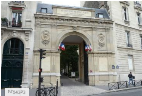
Centre Malesherbes - Central yard
