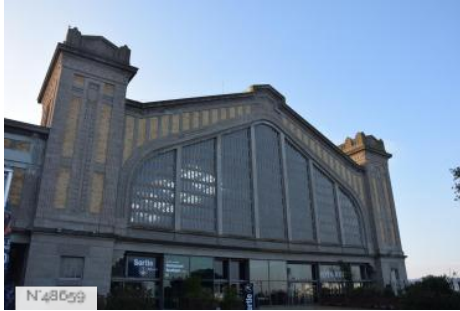
N 48059 Cité de la Mer Museum - Old Transatlantic Maritime Station
