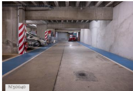
Centre National de la Danse Parking
