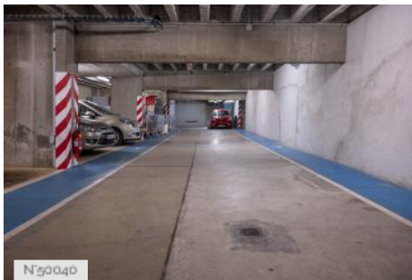
Centre National de la Danse Parking
