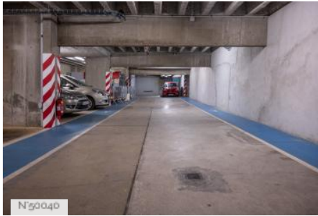
Centre National de la Danse Parking
