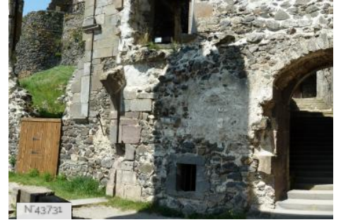
Castle of Murol - Courtyard access
