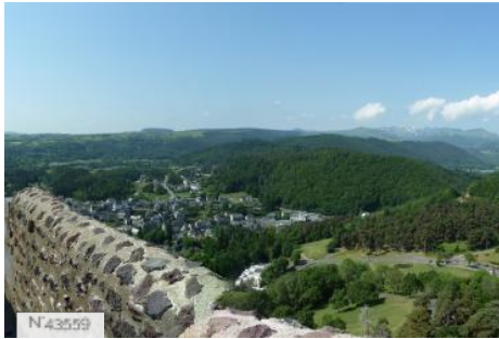
Muroi castle - Tower and covered way
