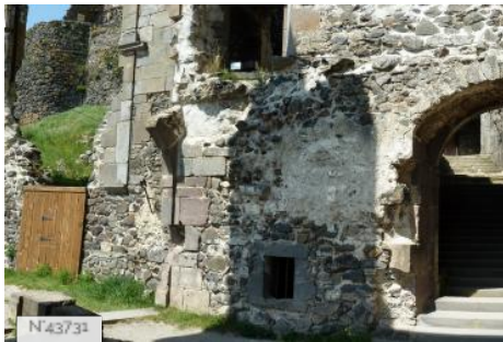
Castle of Muroi - Courtyard access
