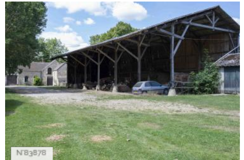
N83878 Château de Nandy - Grange
