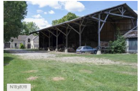
N83878 Château de Nandy - Grange
