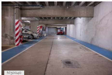
Centre National de la Danse - Parking
