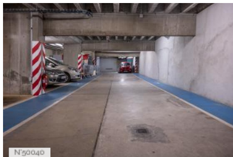
Centre National de la Danse - Parking
