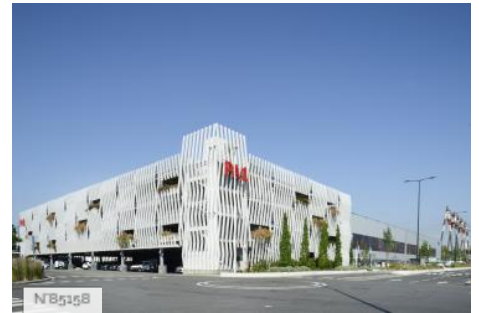
N85158 Marché International de Rungis - Parking silo
